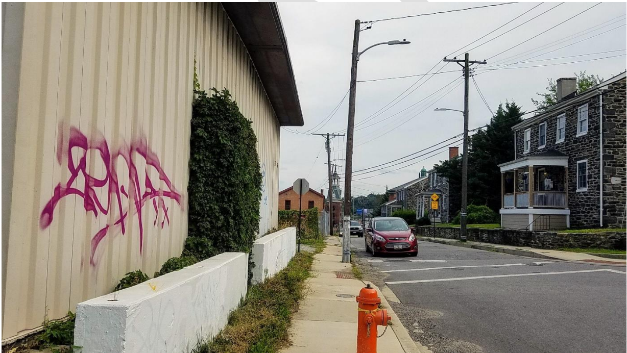
Image 17: 3535 Clipper Road, left, looking south, August 27, 2020
